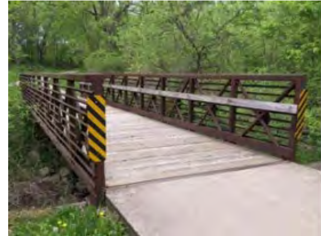
An example of wood decking - CSA S7 Section 2
