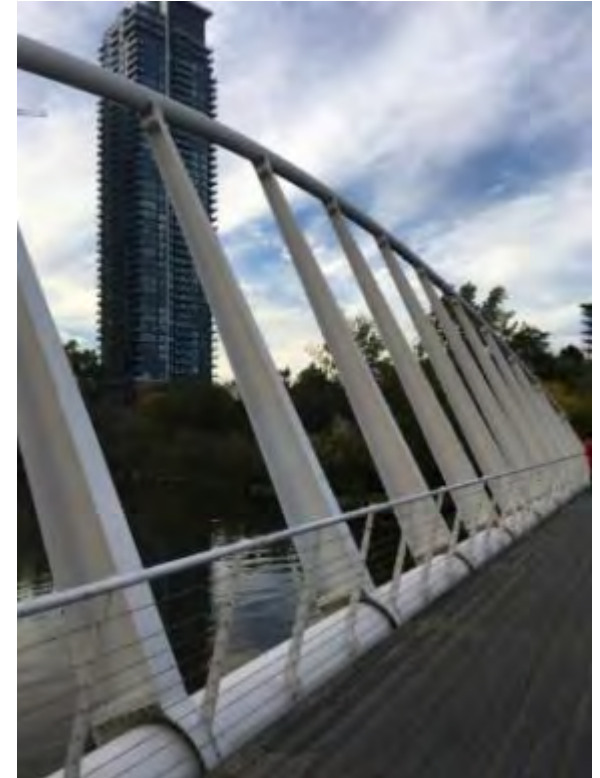
Mimico Bridge, Toronto – CSA S7 Annex B
