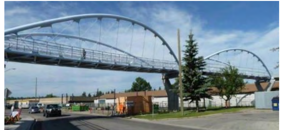
Pottery Road Bridge, Toronto – CSA S7 Annex B
