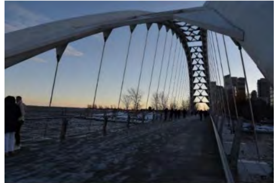
Humber Bridge, Toronto, ON – CSA S7 Annex B
