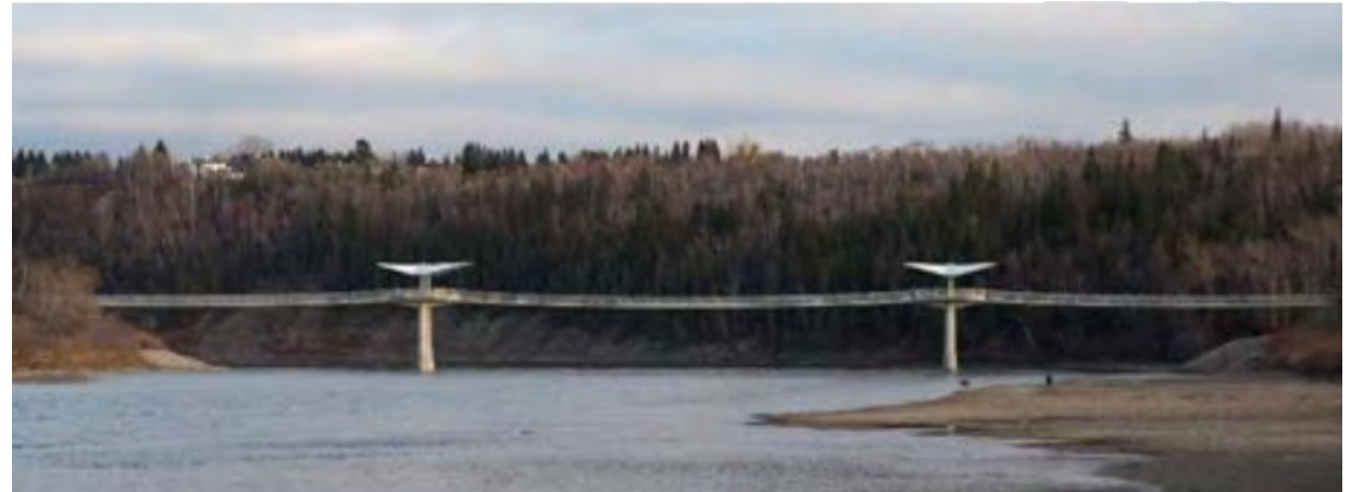
Terwillegar Bridge, Edmonton – CSA S7 Annex B
