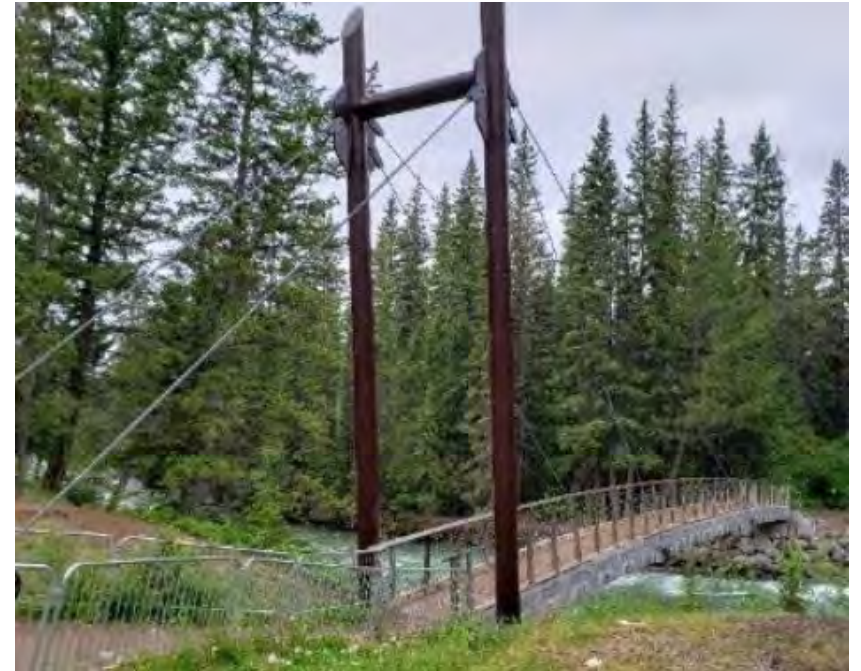
Fifth Bridge, Jasper, AB, Cable stay footbridge with gluelam timber girders – CSA S7 Annex B
