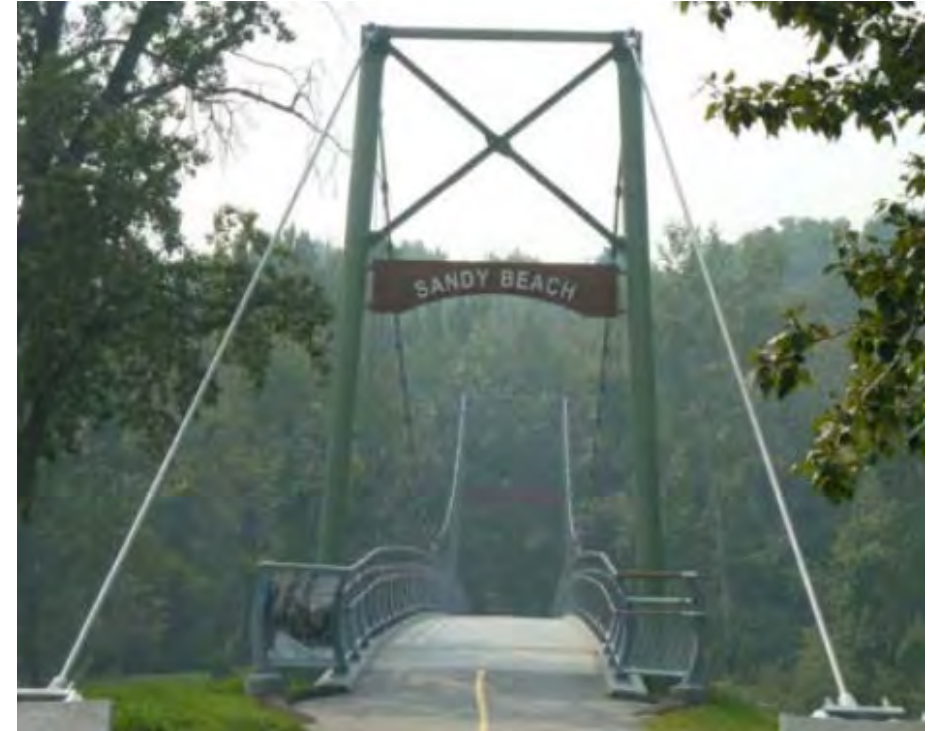
Bridge over Elbow River, AB – CSA S7 Annex B
